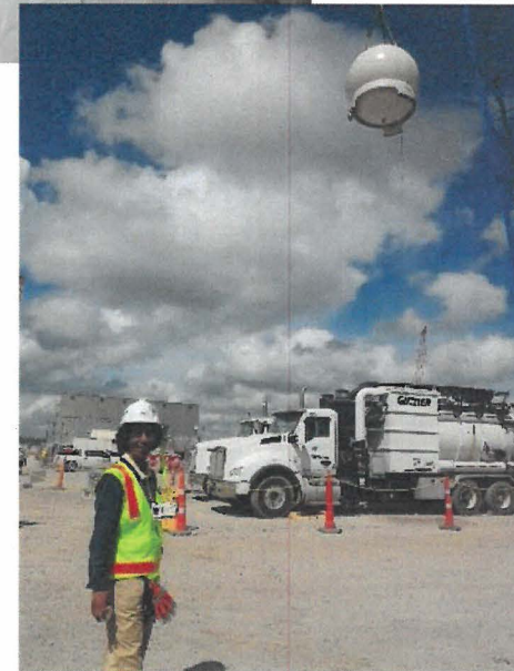
NRC inspector observing Unit 4 accumulator lift
