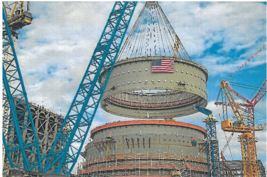
Installation of Ring 3 on Vogtle Unit 3 Source: Southern Nuclear Company
