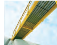
Gangway for the chemical industry
