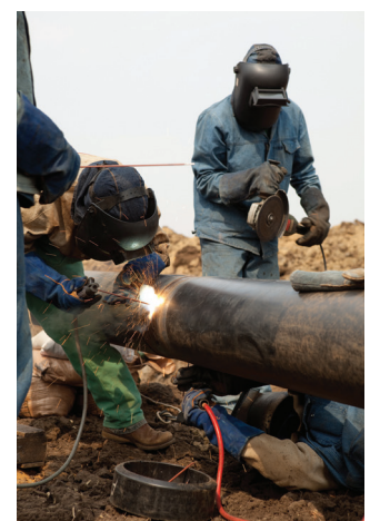
Pipeline Construction/ Maintenance
