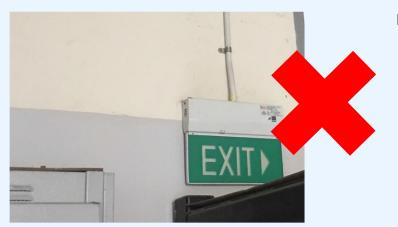
Exit Sign not in efficient working order e.g. not illuminated when the test button is depressed
