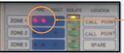
Isolation / Fault showing at fire alarm panel should be investigated promptly and be rectified
