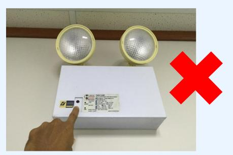
Emergency light not in efficient working order e.g. not illuminated when the test button is depressed
