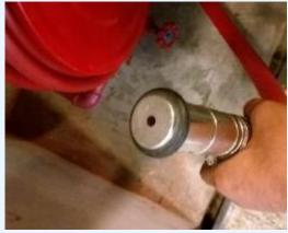
Hosereel is tested regularly with adequate throwing distance (i.e. jet discharge of at least *6m*)
