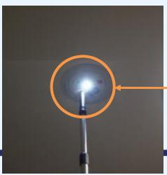
Emergency lights is efficient working order when it is lit when the "test" button is depressed.
