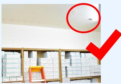
Sprinkler head should not be obstructed (i.e. at least 0.5m unobstructed)
