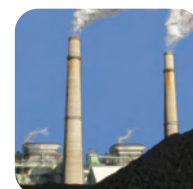
Coal-fired power plant emissions
