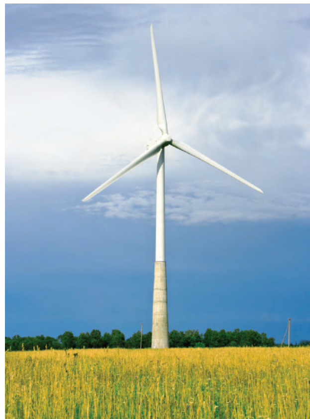
Figure 2-10 Kinetic energy, created by the gaseous molecules in a mass of moving air, turns the blades of this wind turbine. The turbine then converts this kinetic energy to electrical energy, which is another form of kinetic energy.
