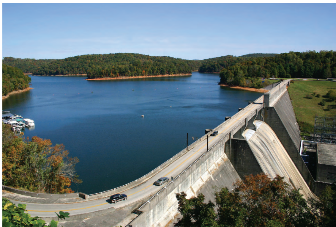
Figure 2-12 The water stored in this reservoir behind a dam in the U.S. state of Tennessee has potential energy, which becomes kinetic energy when the water flows through channels built into the dam where it spins a turbine and produces electricity—another form of kinetic energy.
