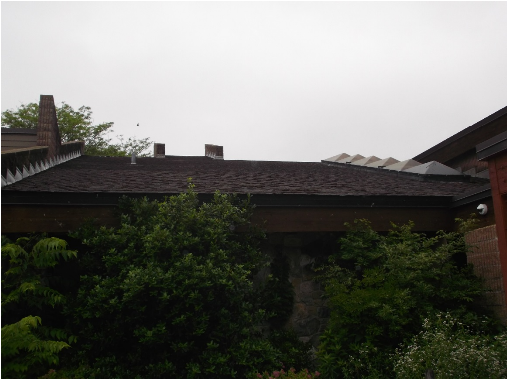
EXHIBIT 'D' ADMINISTRATION ROOF / SKY LIGHT
