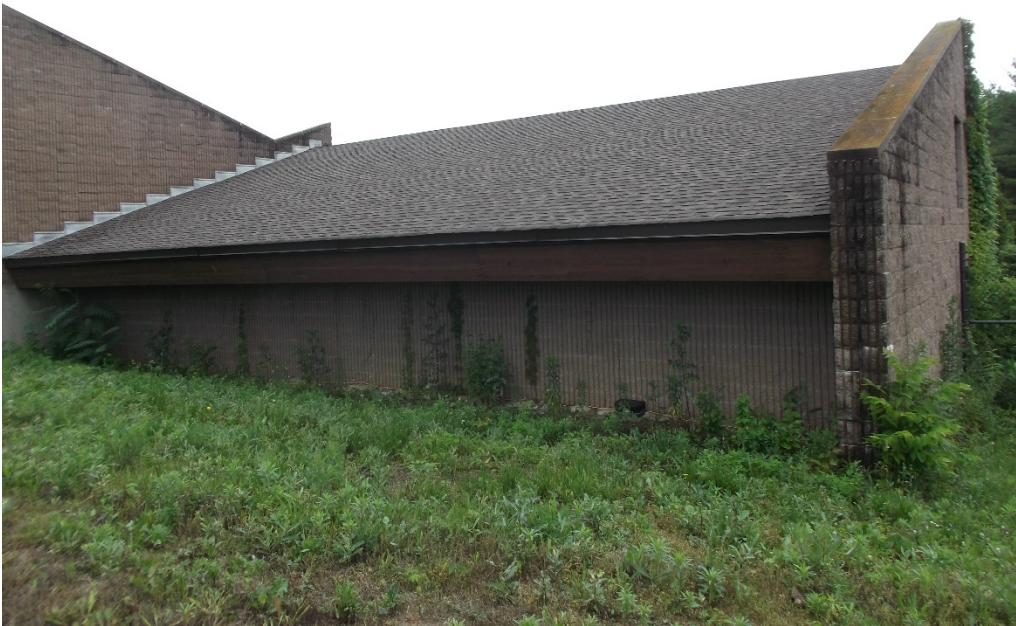
EXHIBIT 'D' ADMINISTRATION BUILDING ROOF
