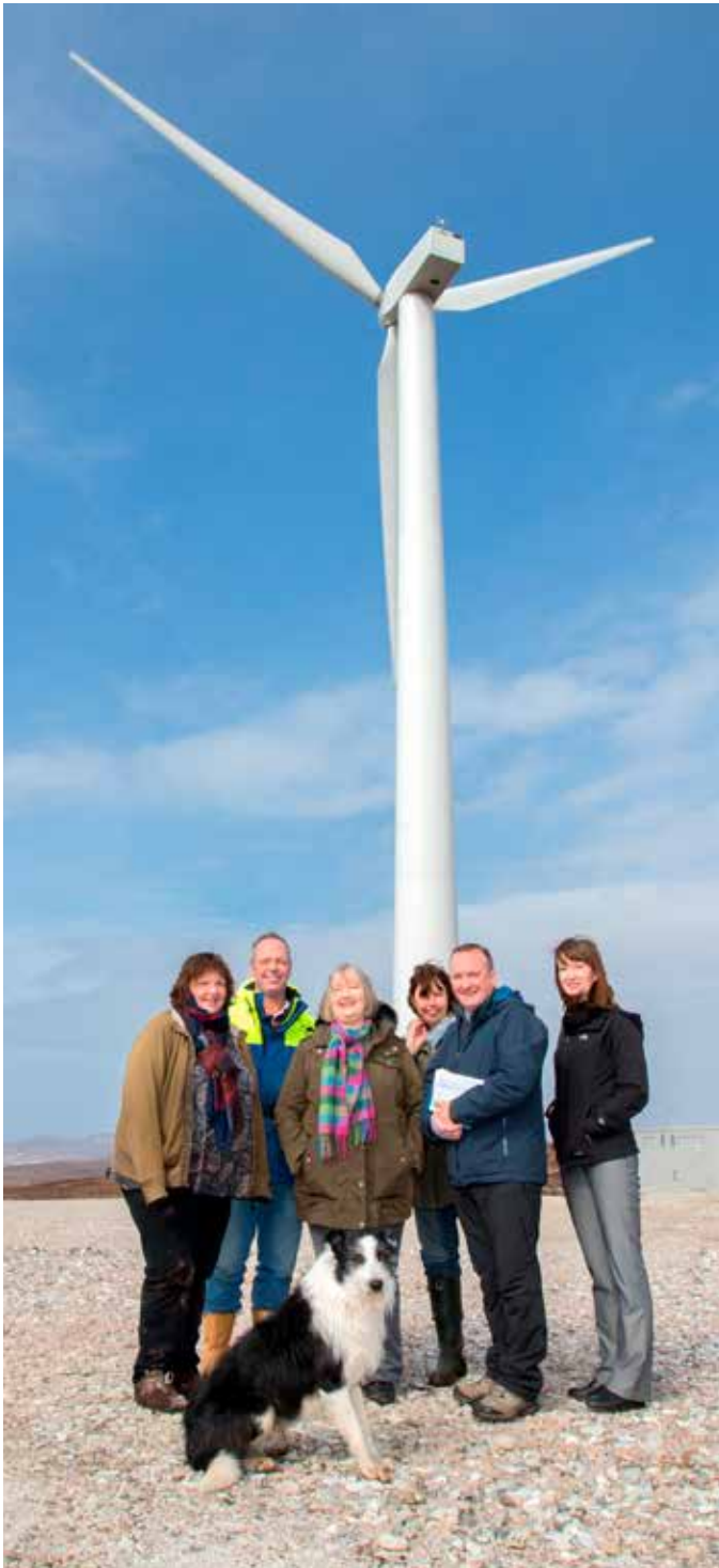
Coigach Community Wind Turbine (Credit: Highlands and Islands Enterprise)
