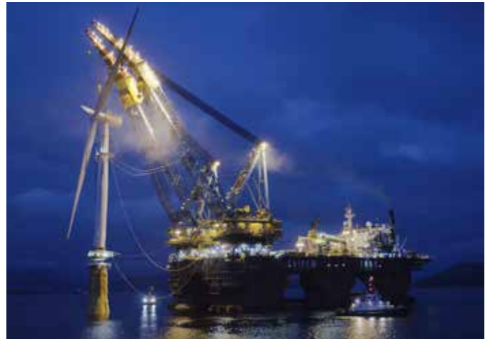
Hywind Scotland Pilot Park construction (Credit: Roar Lindefjeld, Statoil)
