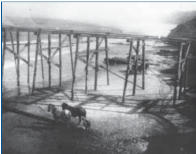
Snaking piles for the first pier construction, 1916. Logs were offloaded from ships from Los Angeles, then floated ashore. The original wooden pier stood until replaced in 1988.
