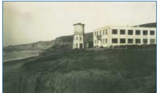
The “Saltwater Tower” and the George H. Scripps Building, ca. 1910, the first buildings on the present day site. The Saltwater Tower was demolished in 1932. The Old Scripps Building today houses the graduate student office and a classroom.
