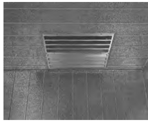
The evaporator section mounts flush in the standard 4"-thick ceiling panel.
