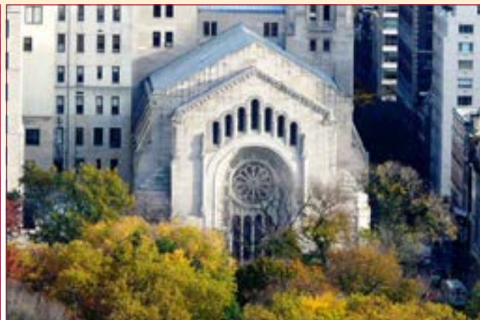
The current historic sanctuary at Fifth Avenue and 65th Street was completed in 1929 and has been our home for over 90 years.
