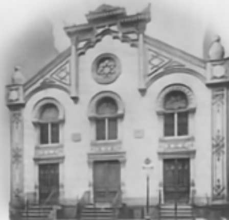
In 1847, Temple Emanu-El moved north to a church on Chrystie Street, which was then rededicated.
