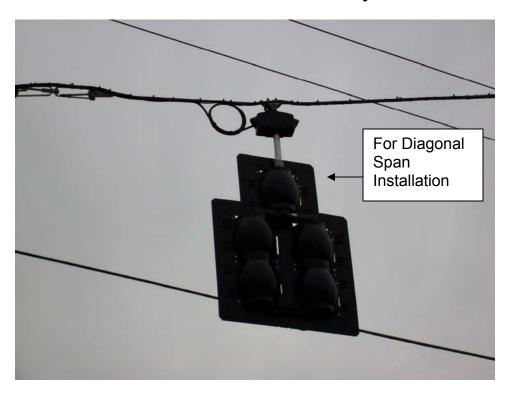
If the single point is a box span, individual NEMA enclosures (junction boxes) will be mounted on each strain pole and individual signal cables run from the NEMA enclosures (junction box) to each signal. For box span installation and certain diagonal spans, the disconnect will be eliminated. Below is attachment criteria.
