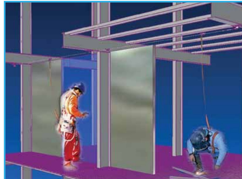
Intermediate Anchor With By-Pass Bracket
