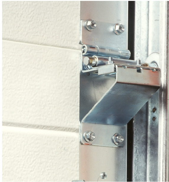
Figure 22: Hinge with roller bracket and roller [3]
