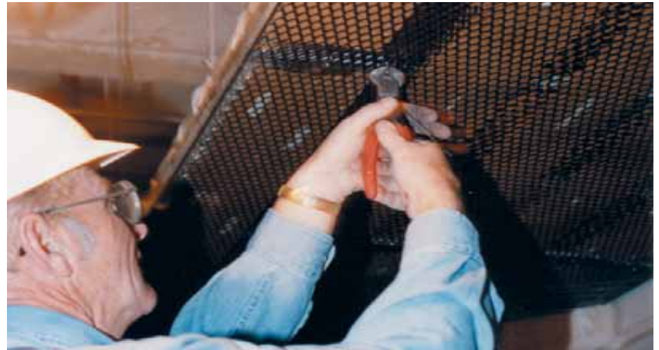
SECURA LATH INSTALLATION for Direct Application to Framing Members for Wall and Ceiling Installation
