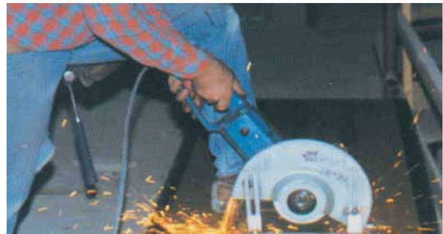
Cutting Secura Lath Sheets
