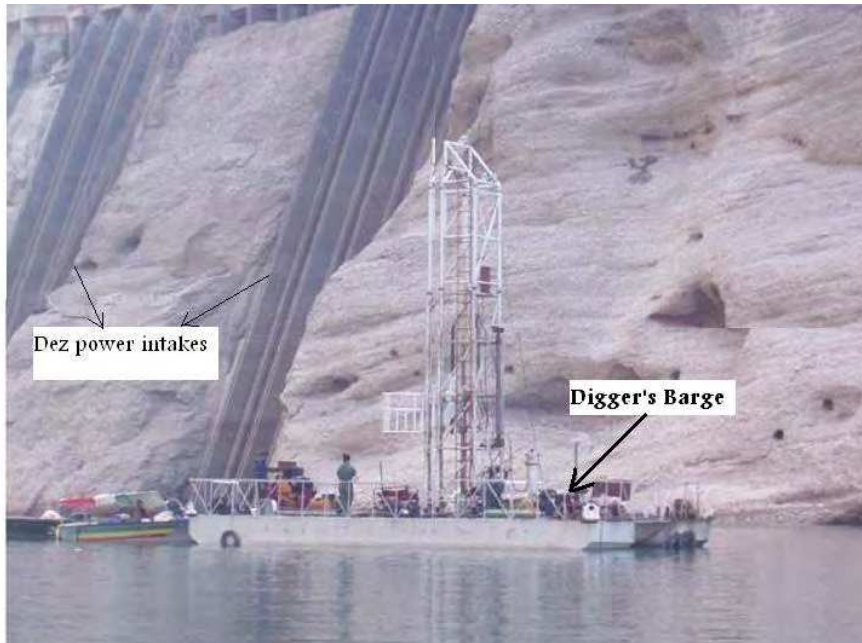
Fig. 3. Photos of barge and digger located near Dez power intakes.
