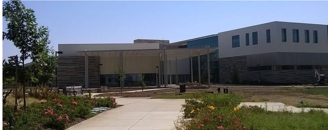
Join us October 13th at 10 a.m. for the grand opening of the Betty Irene Moore Hall and the Retiree Center's Sacramento office.
