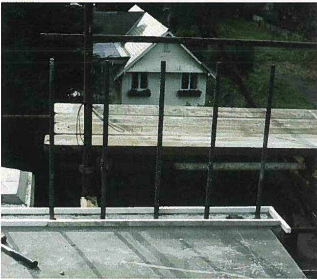
(c) Protruding bars used in wall panel connection
