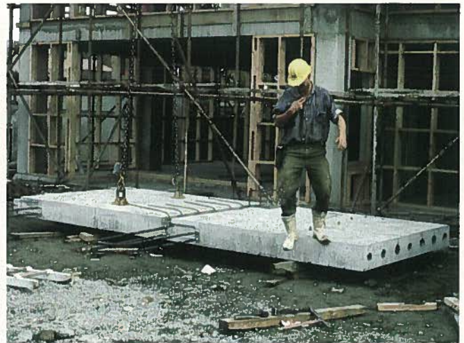
(b) Wall panel before erection
