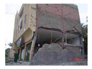
Fig. 13: Unacceptable bracing system, the cross-section of bracing member is insufficient.
