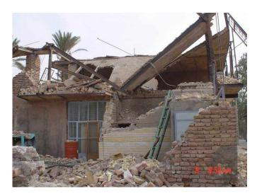
Fig. 10: first group of steel buildings, combination of steel internal columns and load-bearing external brick-walls.
