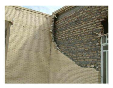
Fig. 9: an example of reinforced brick buildings in the earthquake-affected area with a relatively good performance.
