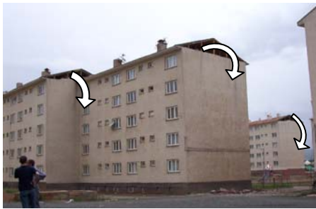
(a) Falling of gable walls caused broking about 20 cars
