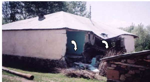
Figure 11 A view of load bearing walls collapsed in the out-of-plane direction during Bingöl Earthquake
