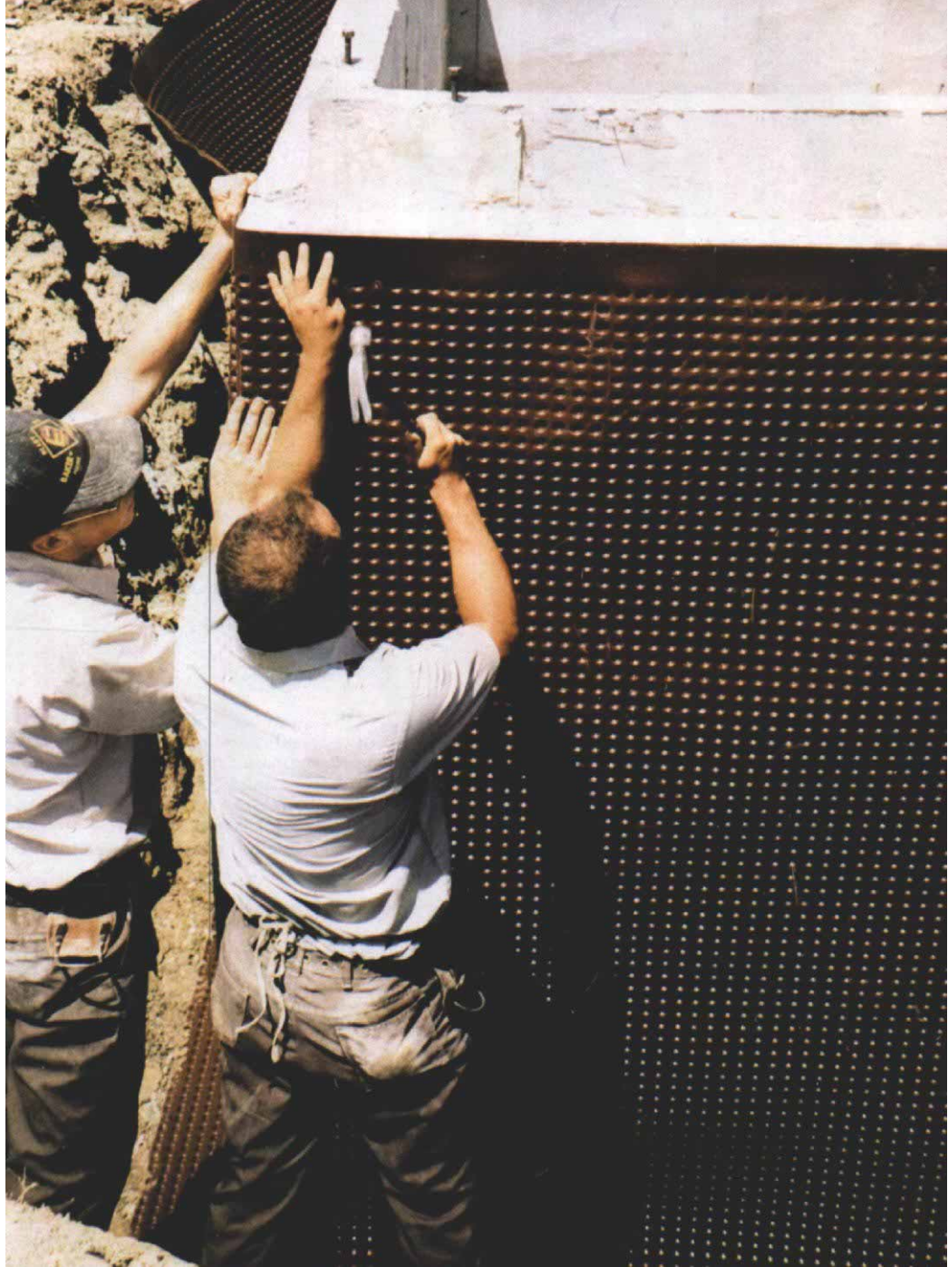
Dimple sheeting provides drainage. This polyethylene sheeting resists moisture while the dimples provide air gaps that channel away any groundwater that might get through. Photo by Brent Anderson.
