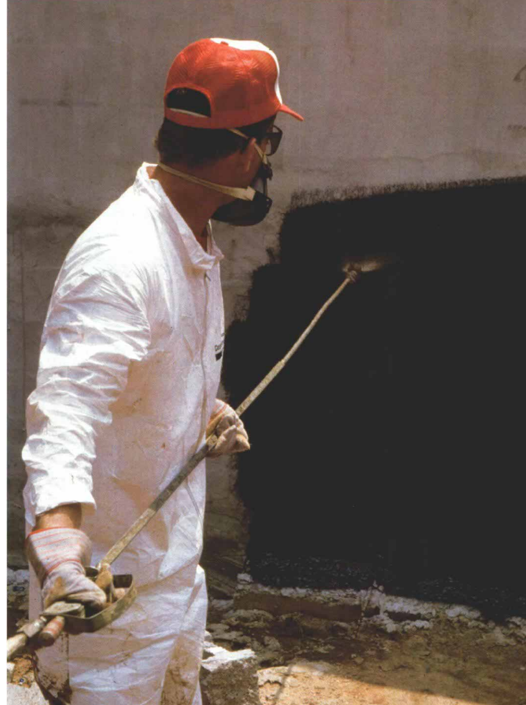
Liquid-applied membranes are usually sprayed on. Liquid-applied polymer-modified asphalts such as Koch's Tuff-N-Dri emulsion cure to form seamless, self-flashing waterproof membranes over concrete or masonry. Photo courtesy Koch Materials Company.
