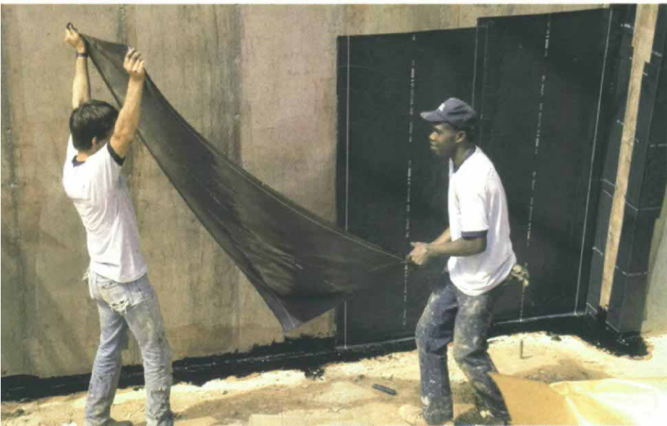
Peel-and-stick membranes stretch to bridge cracks. Self-adhering rubberized asphalt membranes such as W. R. Grace's Bituthene withstand tremendous hydrostatic pressure and can be backfilled immediately. Joints between footings and walls are covered with mastic or mortar for durability. Photo courtesy W. R. Grace & Company.
