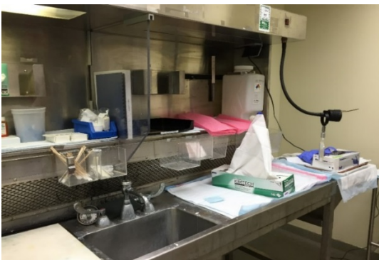
Figure 32 Ventilated Wet Bench
