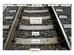
Fig. 1. Definition of basic track elements.
