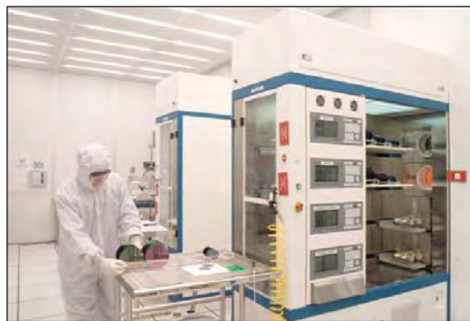
Figure 2. Oxidation and annealing furnace banks.
