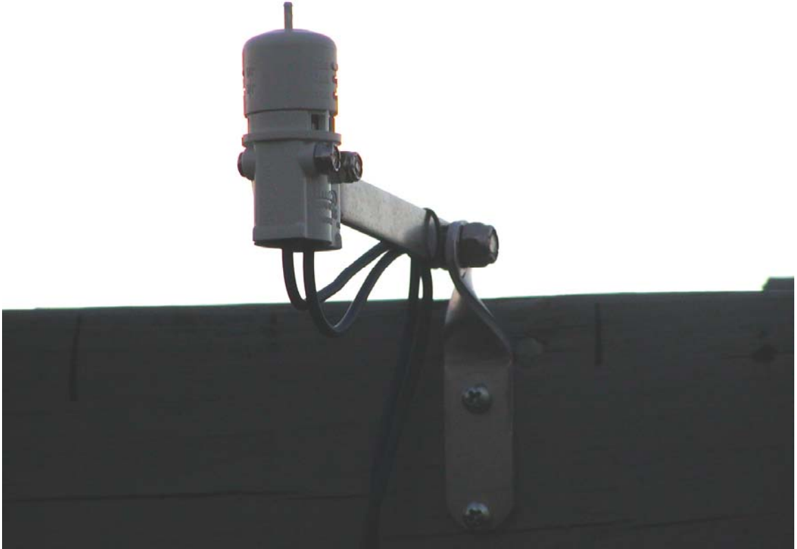
Figure 2-4. Rain sensor installed for this study.
