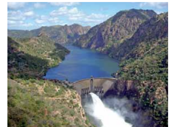
Cahora Bassa HPP (courtesy of Hidroelectrica de Cahora Bassa)
