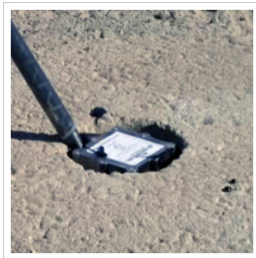
Figure 4.13. Filling hole with epoxy until level with road surface
