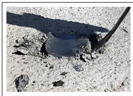
Figure 5.7. Prying upward on opposing side
