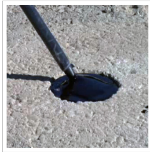
Figure 4.14. Filling hole with epoxy until level with road surface
