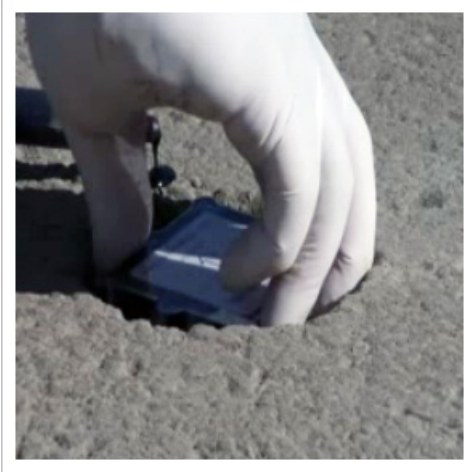
Figure 4.12. Placing the sensor in road
