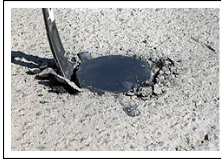
Figure 5.4. Prying upward to loosen shell top
