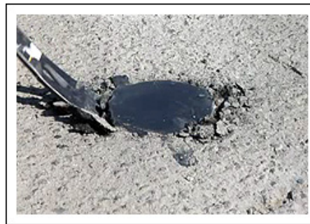
Figure 5.5. Prying upward to loosen shell top
