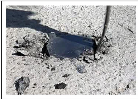
Figure 5.6. Prying upward on opposing side
