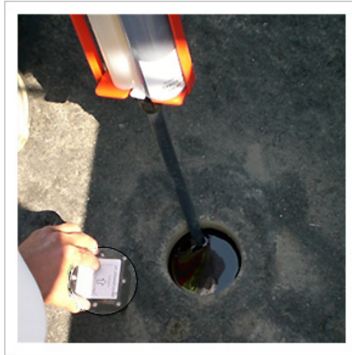
Figure 4.11. First epoxy application
