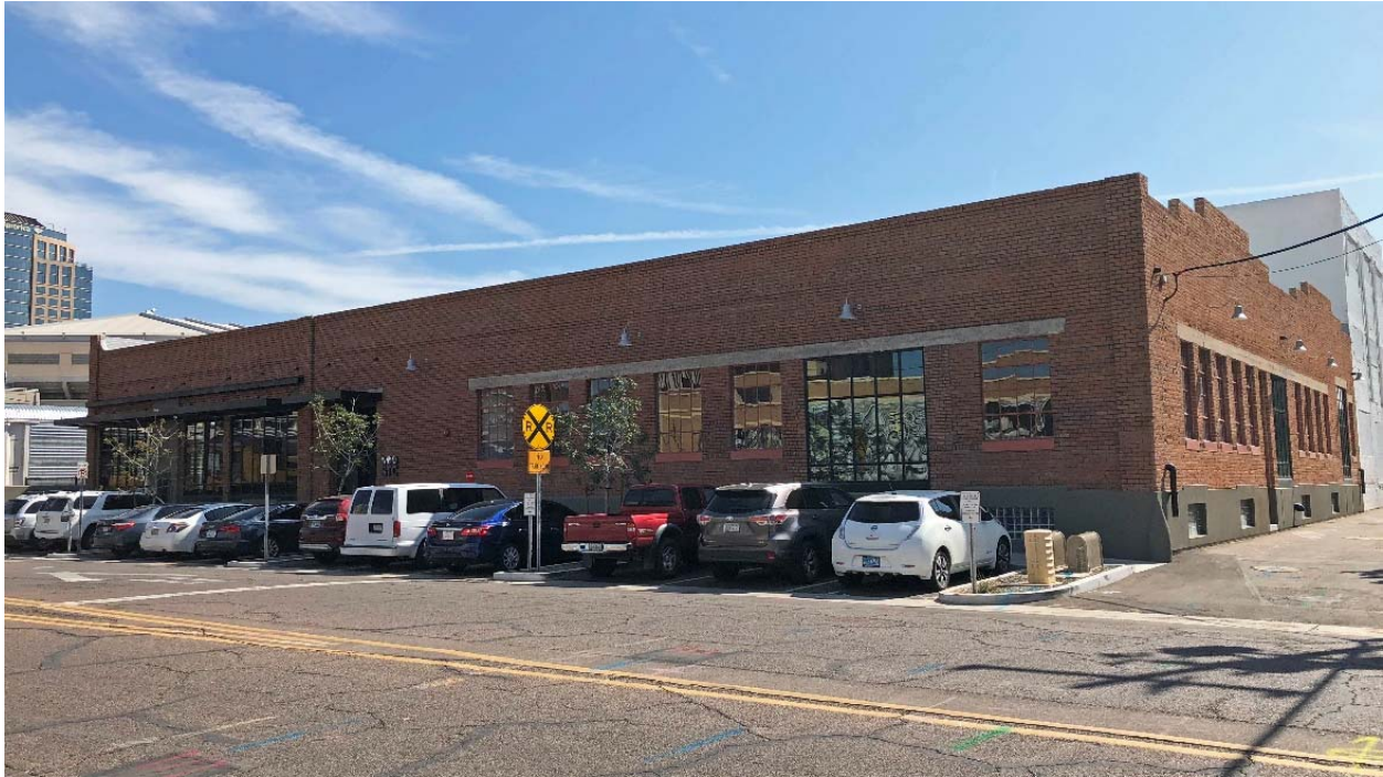
Photo 5. View of west façade after rehabilitation, facing northeast (2018).
