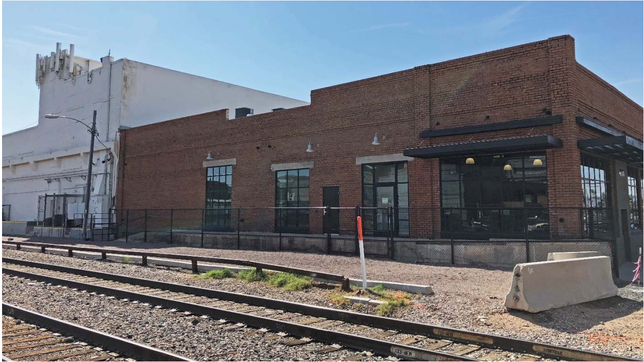
Photo 7. View of north façade after rehabilitation, facing southeast (2018).
