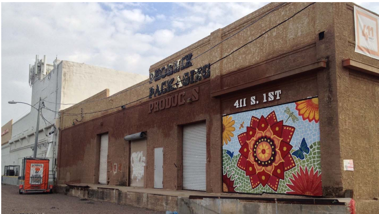
Photo 2. View of north façade prior to rehabilitation, facing southeast (2016).
