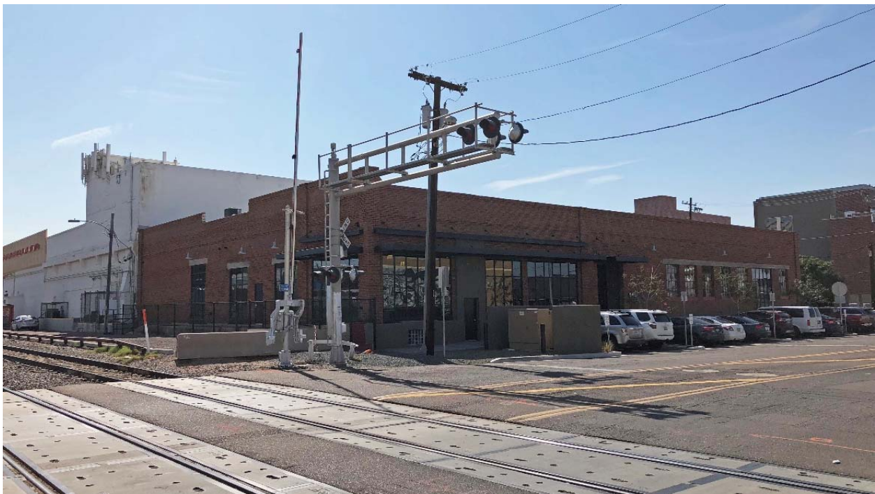
Photo 6. View of west façade after rehabilitation, facing southeast (2018).
