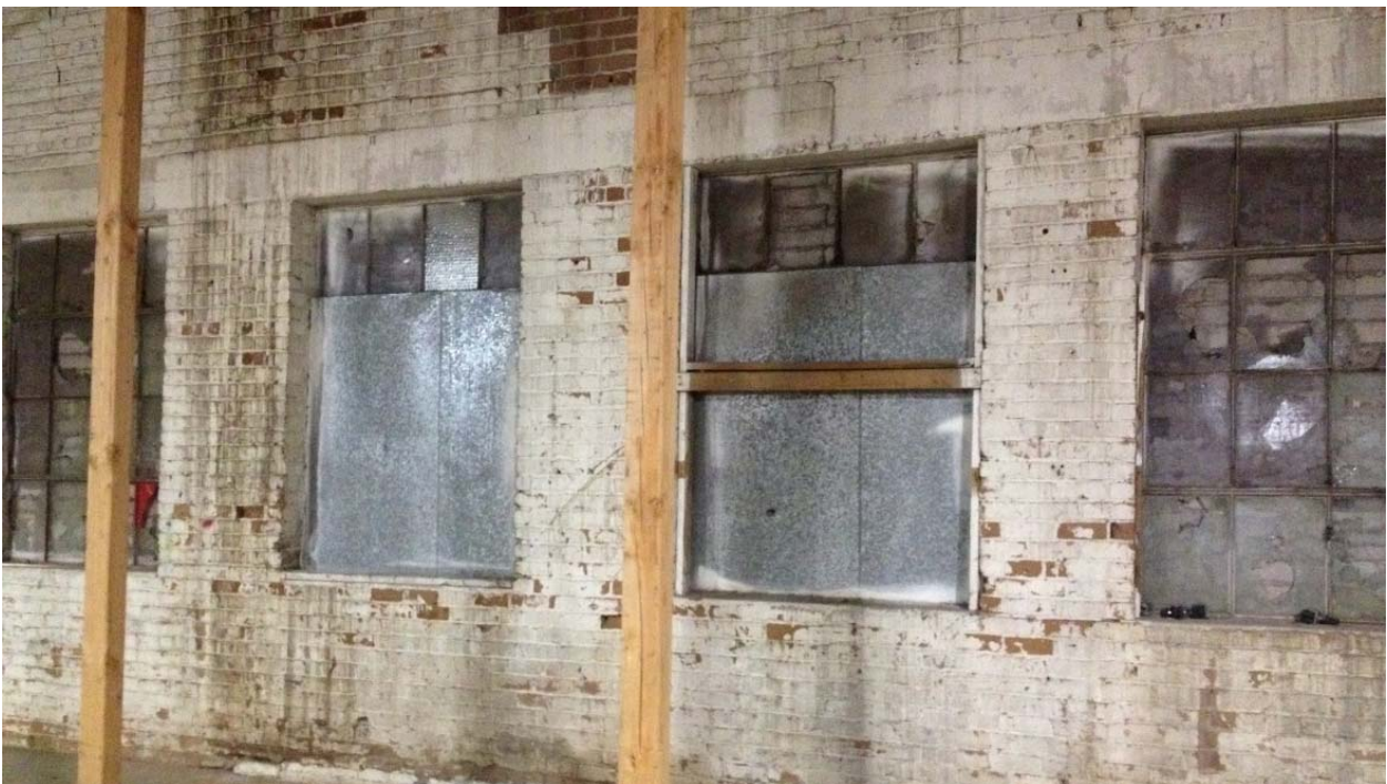
Photo 4. Infilled windows from interior, prior to rehabilitation (2016).
