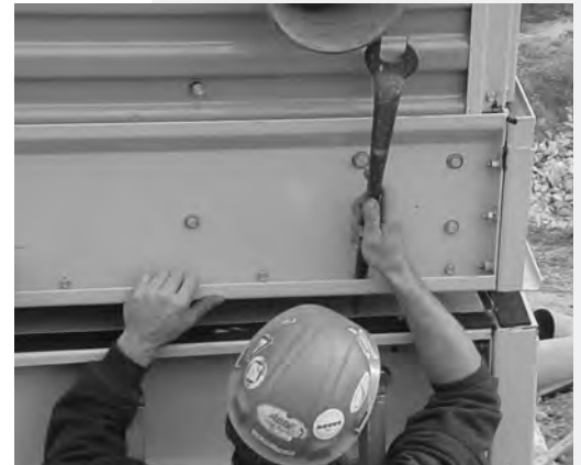
Figure 5. Drift Pin Alignment
