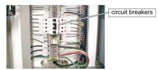
Figure 5-10: Circuit Breakers CB1, CB2 and CB3 Location
