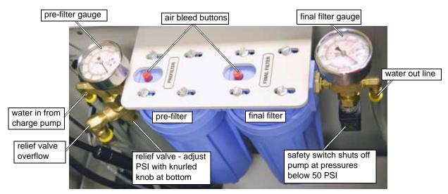
Figure 7-51: Pump Internal Water Filtration System
