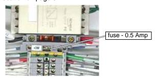
Figure 5-12: 24 VDC Power Supply Fuse Location
