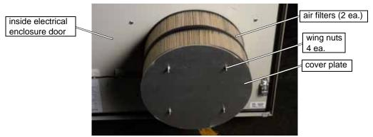
Figure 7-58: Electrical Enclosure Air Filters
