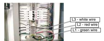
Figure 5-6: AC Power Legs L1, L2, and L3.
