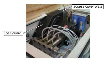
Figure 7-39: Access Cover Plate on Top of Pump Belt Guard
