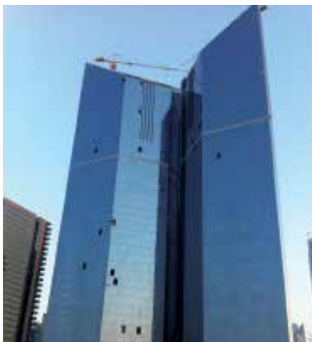
Near Completion Phase
