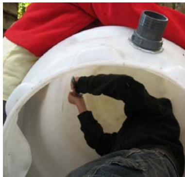
One child tightens the nut from inside the barrel while another holds the spigot on the outside.
