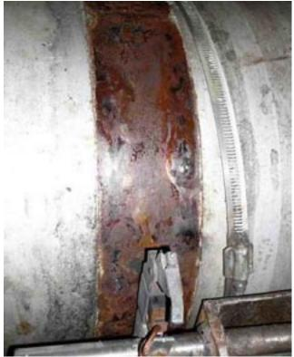
Corrosion hiding behind the slip ring
