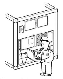
PC connected to the communication port
