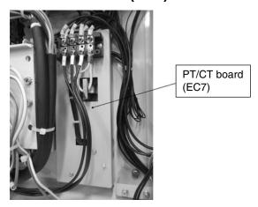
This printed circuit board has the two functions as a measuring instrument and protective device and provide as an interface between the main circuit (high voltage) and controller.
