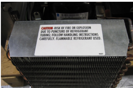
CONDENSER COIL SHROUD
