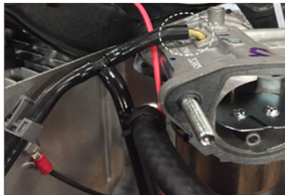
Figure 3. New T-Fitting/Line Assembly Installed.
