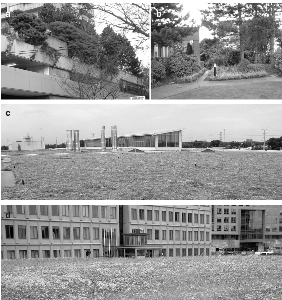
Figure 1. Examples of (a, b) intensive green roofs (with deeper substrate, more elaborate vegetation, and higher maintenance requirements) and (c, d) extensive green roofs (with shallow substrate; hardy, drought-tolerant vegetation; and low maintenance requirements). Photographs: Brad Rowe.
