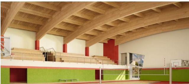
Wooden beams as support for the wooden roof of the gym
