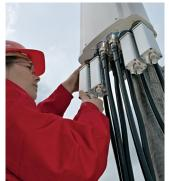
After feederline installation, the optional remote control units (RCUs) can be mounted.
