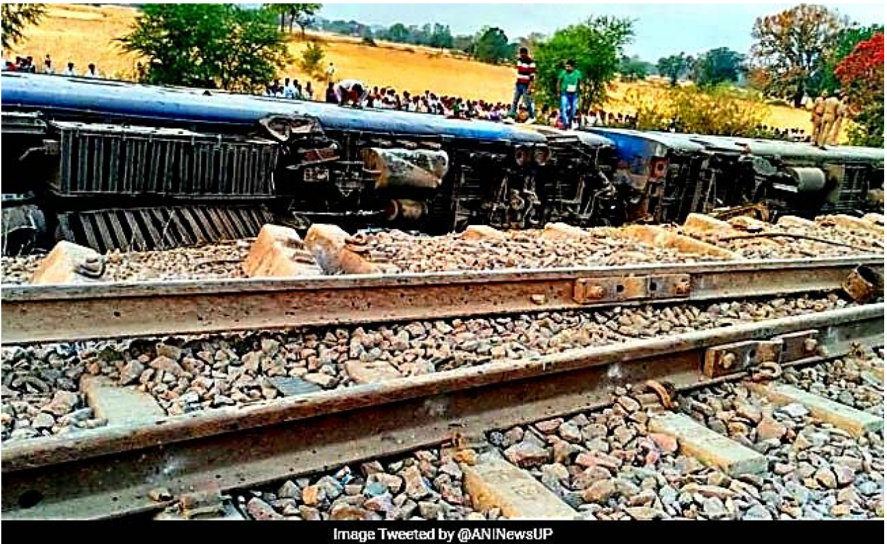
Mahakaushal Express Derailment Spot, 30 th March 2017. Obviously the Quality of the neglected Track did not match the Traffic Load.
