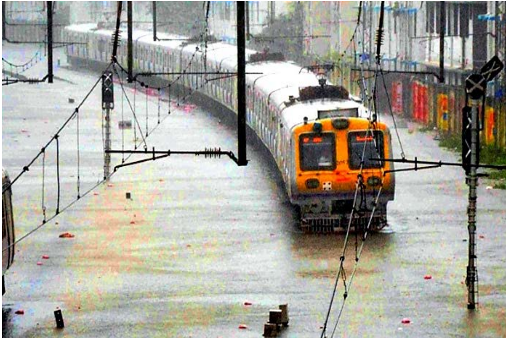
Flooding of Tracks, inadequate City Drainage and Surface Water Management
