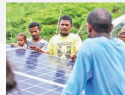
An Aeta community leader orients Sitio Settler residents on the proper operation and maintenance of their solar PV system.
