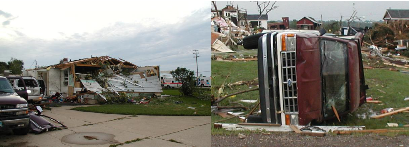
Wall and roof damage to a home, and an overturned van. Note the piece of wood sticking out of the windshield.
