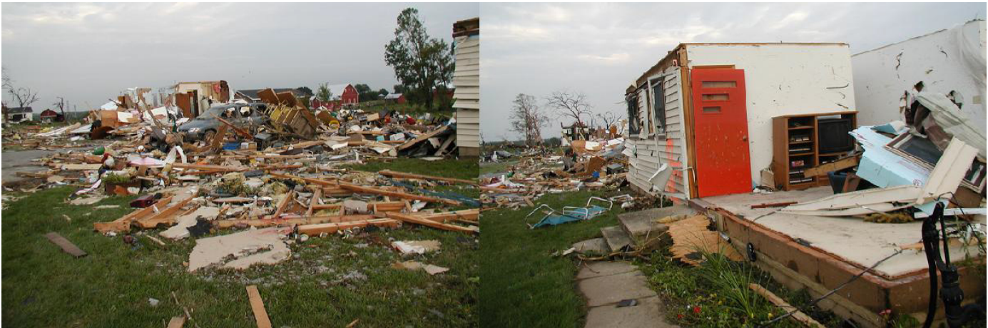
Destroyed homes, blown apart by the winds of the strongest Michigan tornado in ten years.
