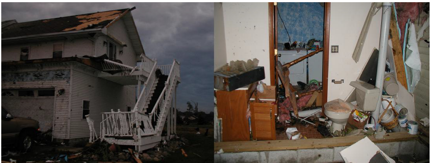
A house and exterior stairs that were battered by the tornado's debris-laden winds, and the inside of a home that sustained heavy damage.
