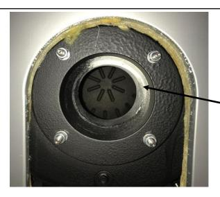
Refractory must be trimmed to fit specific burner
