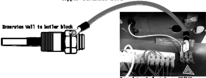
Ground terminal strip on SG/840 Boiler Centrol
