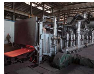
Heating furnace by natural gas
