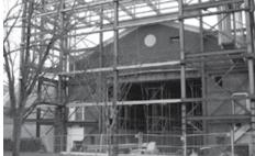
A new back wall that is thirty feet higher than the original has been added, along with new 2008-09 construction on the side to accommodate dressing rooms, a multipurpose staging room and a green room.
