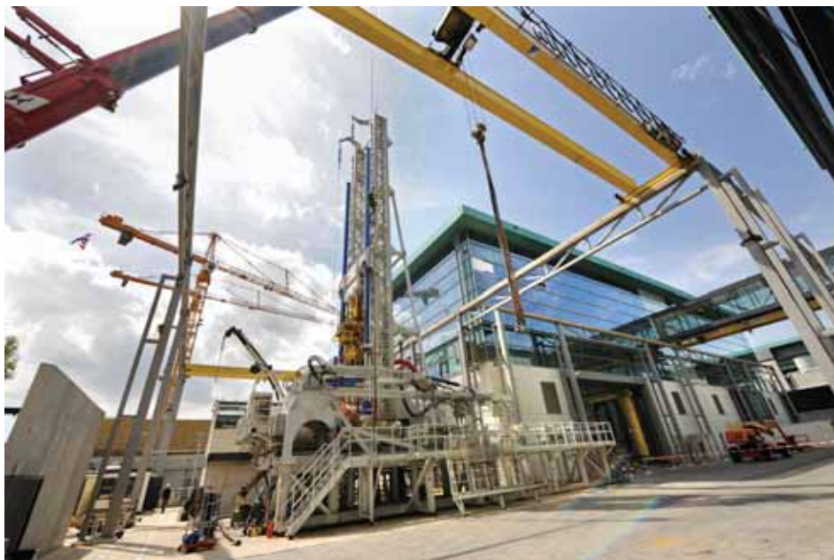
Shell has a 250 ton outdoor drill rig, used to test well construction techniques, new drilling techniques and smart well technologies in field conditions, as well as for training staff on new technologies.
