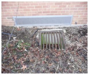
Figure A7. Debris in shallow dry well near outdoor air intake for classroom. Photo by NIOSH.
