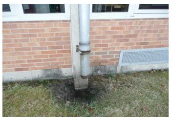
Figure A6. Broken and disconnected exterior roof drain outside classroom. Photo by NIOSH.
