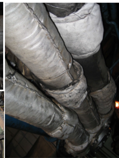
Damaged insulation in E/R and soot inside electrical panel
