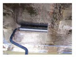
Using a "bubble buster" to roll out trapped bubbles in hand layup laminate [Greg Murphy, Grand Rapids, MI, 2009]
