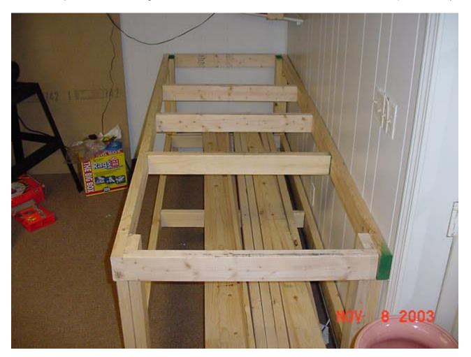
For building the Horizontal Stabilizer and the Vertical Fin (stabilizer), I purchased a 10 foot laminated beam from the lumber yard. It is the flattest straightest surface that would be dimensionally stable that I could come up with. You have to have a 9 foot surface to build the HS, so a 10 foot piece is more than adequate. \$35
