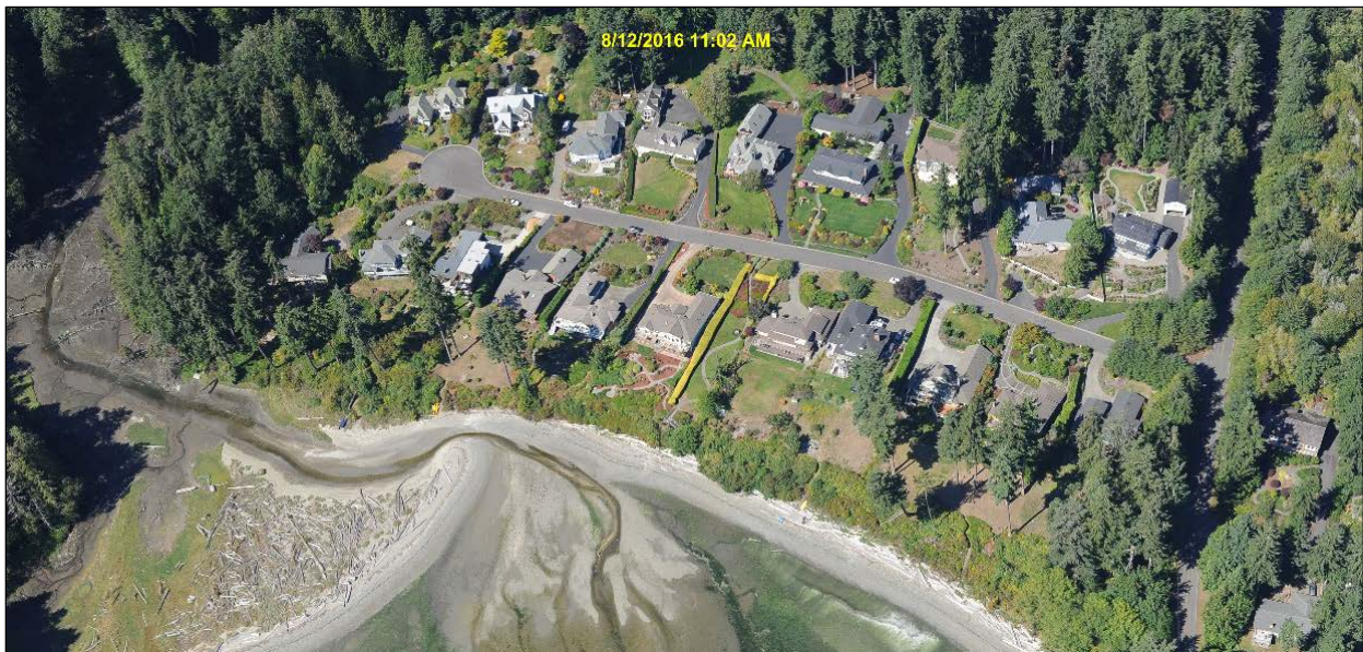
Figure 4-4: Construction of a single-family home by an owner, lessee, or contract purchaser for his or her own use or for family use is exempt from the requirement for a substantial development permit. However, a variance or conditional use permit may be required. (Washington Coastal Atlas photo.)
