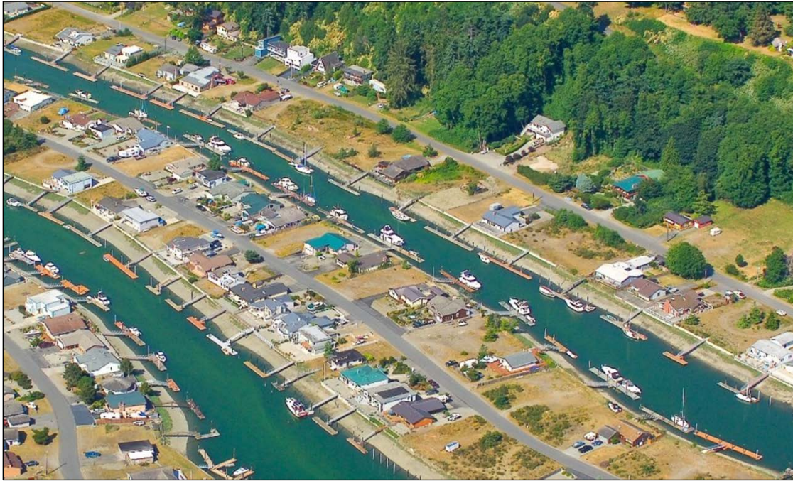
Figure 4-2: Normal protective bulkheads common to single-family residences, such as these in Island County, are exempt from requirements for a substantial development permit. (Washington State Coastal Atlas photo.)
