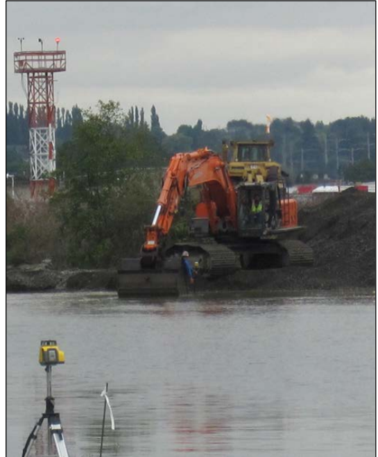
Figure 2-1: Dredging is considered development under the Shoreline Management Act.
